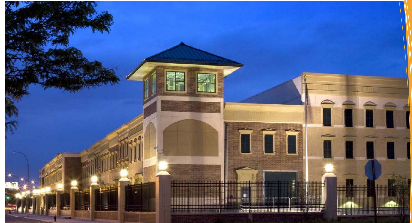
Con Edison, Mott Haven Sub-Station
