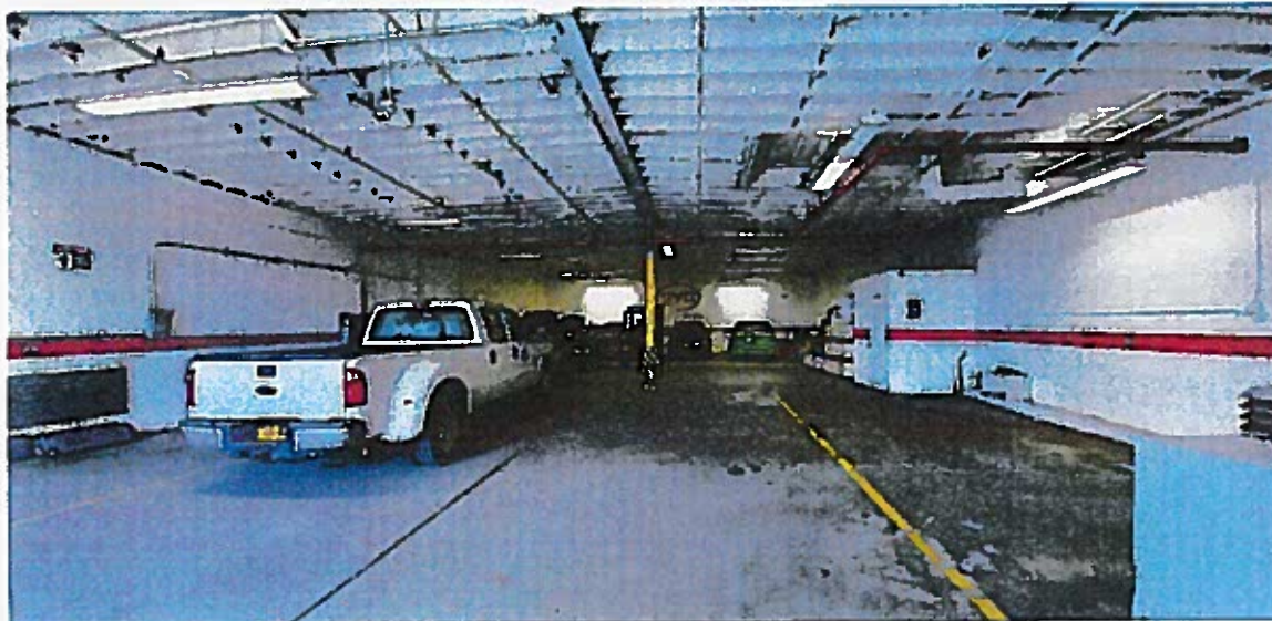
Ground Floor EV Charging Area
