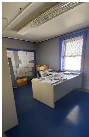
Second Floor Office
