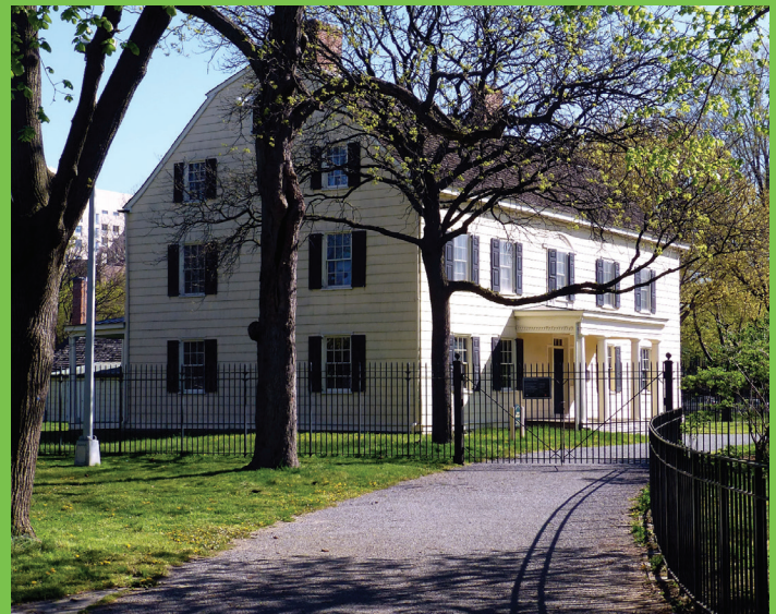
Historic King Manor, which was rehabilitated as part of the Action Plan
