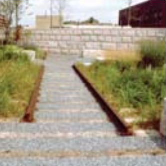
Pervious pavement, Gantry State Park, Queens, NY.
