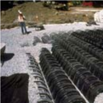
Stormwater detention system under parking lot, Riverdale County School, Bronx, NY
