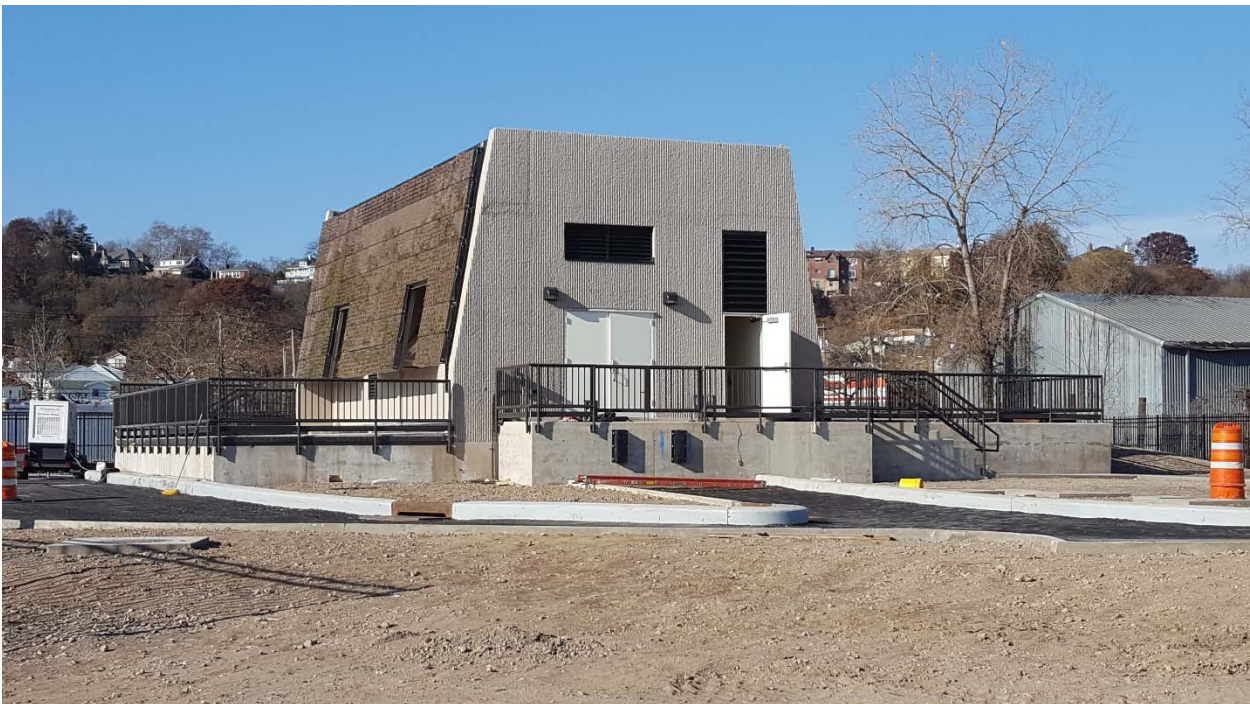
Chlorination Station nears Completion (with newly installed fencing, curbs and driveway)
