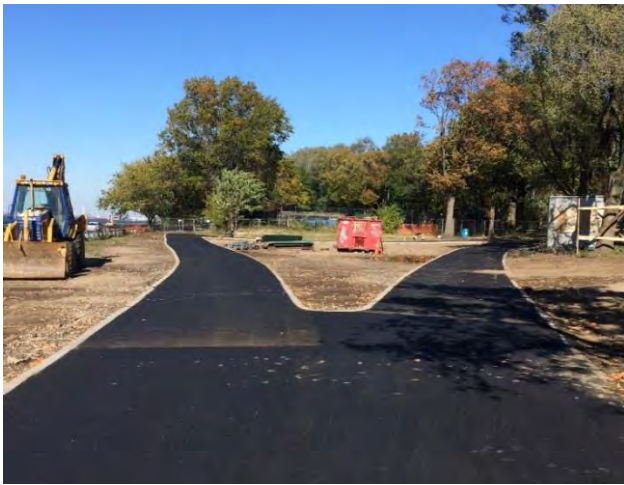
Newly Restored Walking Paths in Shore Road Park
