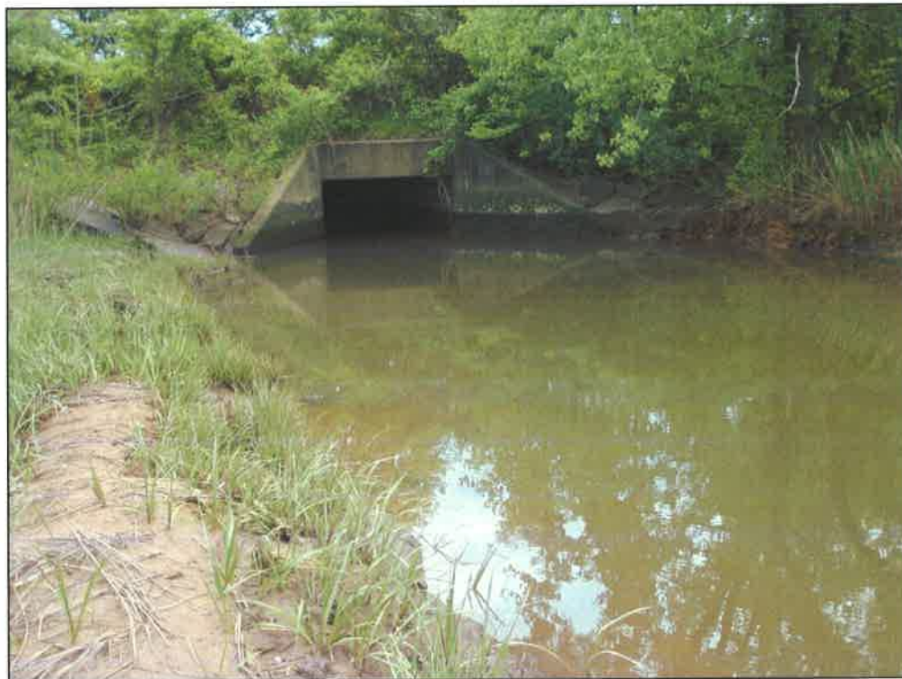
Photo 16: Wetland Flag CH-I1, facing east at culvert under Rt. 440.
