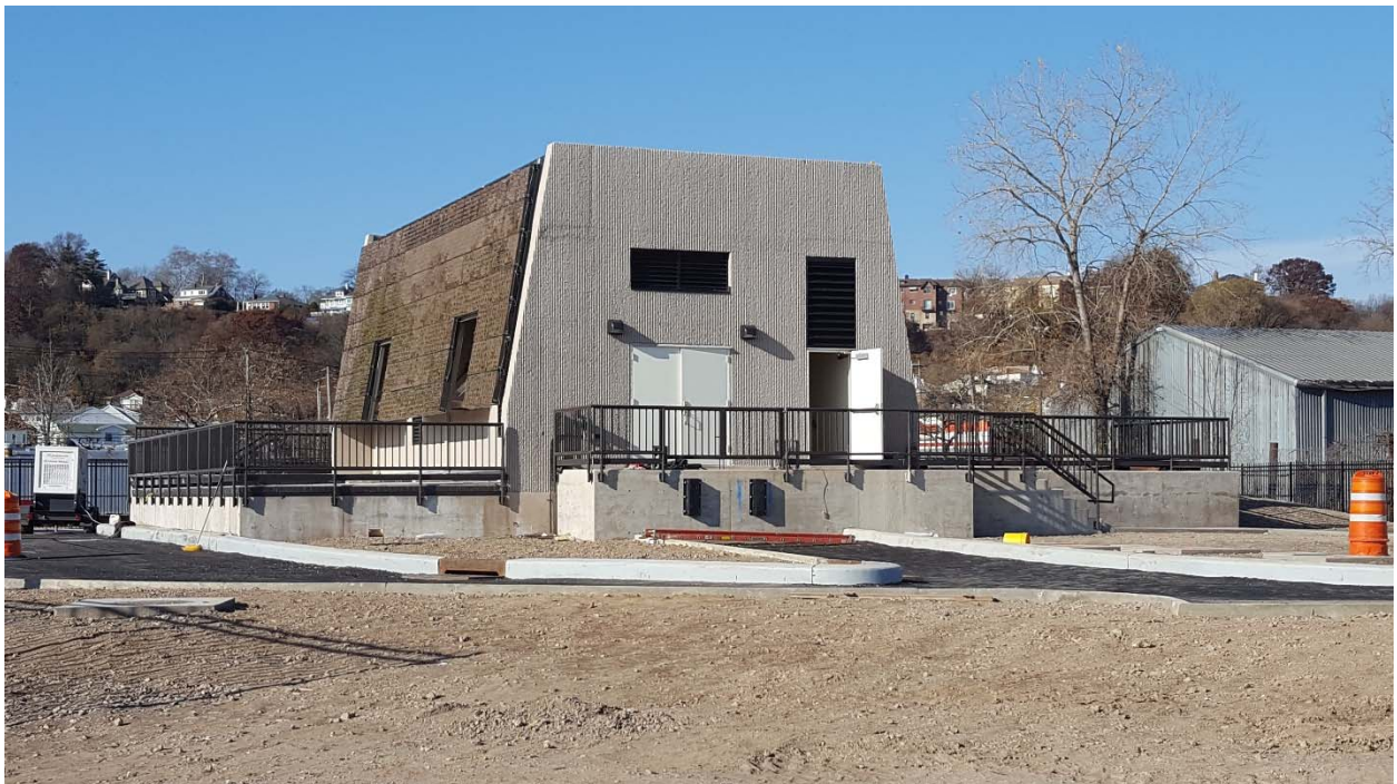
Chlorination Station nears Completion (with newly installed fencing, curbs and driveway)
