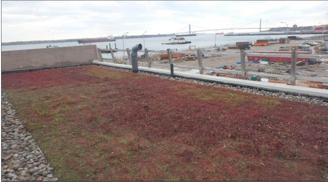
Newly installed Green Roof on top of Chlorination Station. Plants are a variety of Sedum, also known as Stonecrop.
