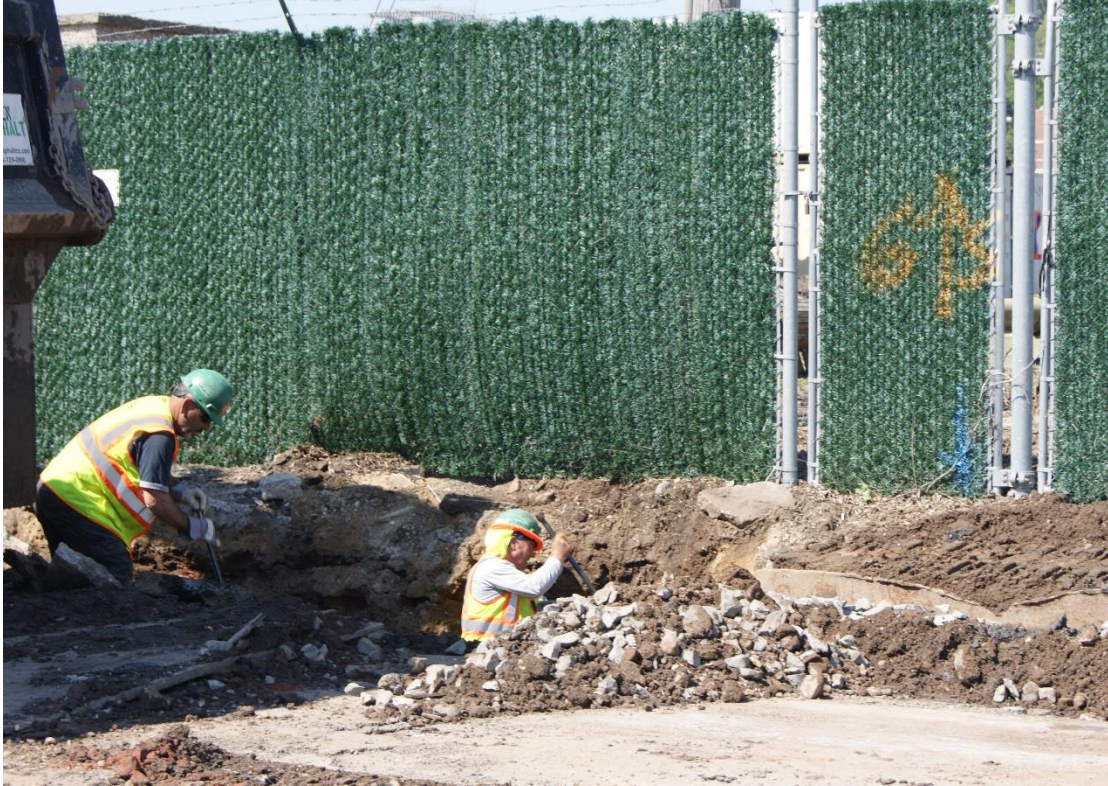
Installation of 18" Sewer along Front Street, vicinity of Richmond Chlorination Station (top and bottom photos)
