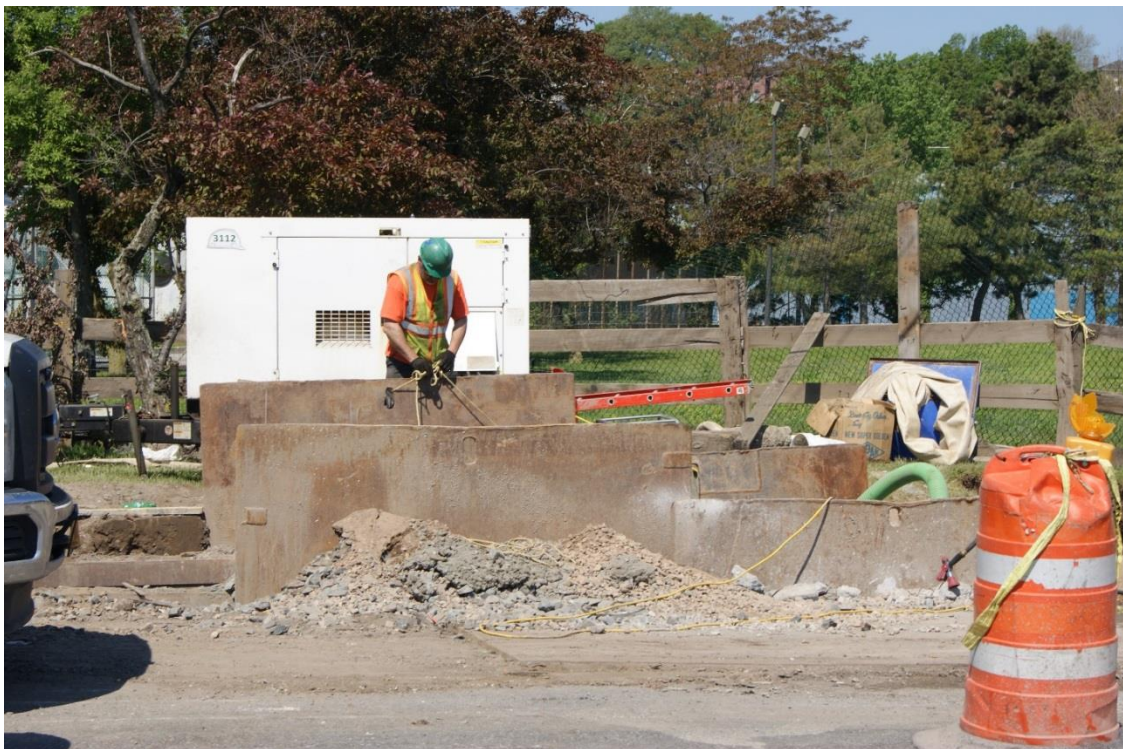
Installation of 18" Sewer along Front Street, vicinity of Richmond Chlorination Station (top and bottom photos)
