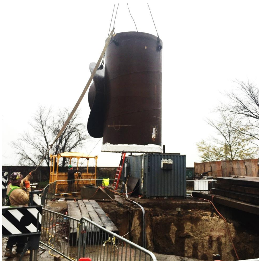
Installation of section of riser pipe at Brooklyn Shaft Site
