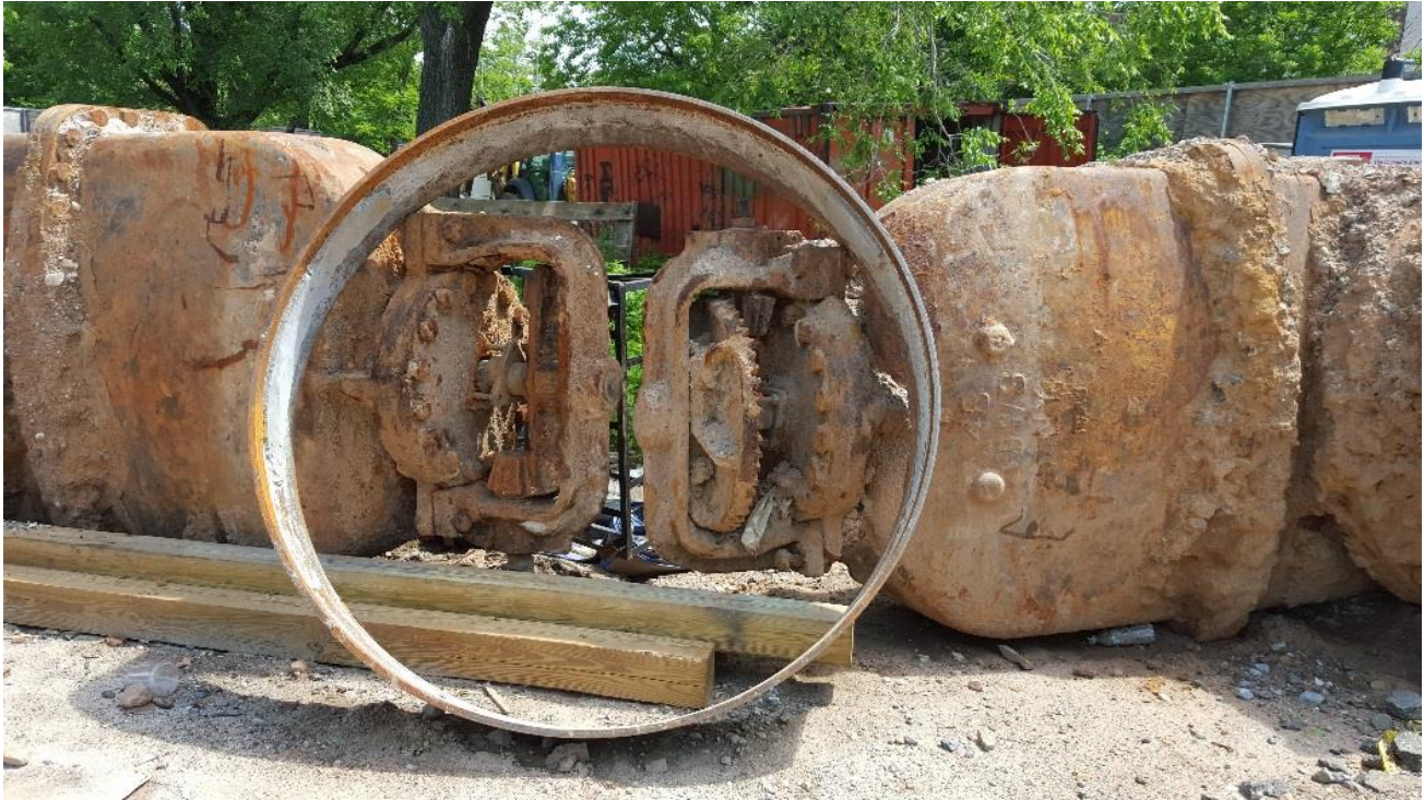
Section of old Siphon Removed from Brooklyn Shaft Site
