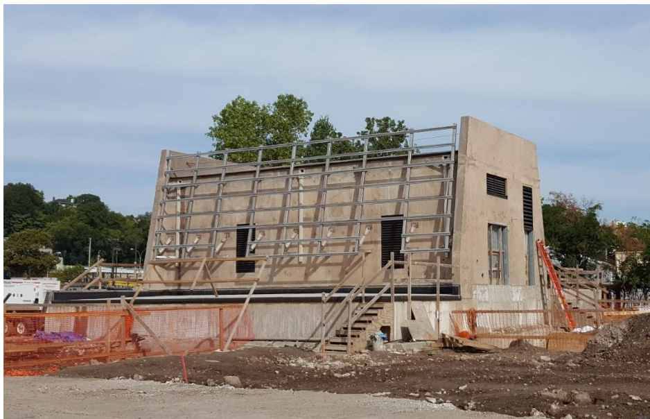
Frame for “Living Wall” begins to take shape on new Chlorination Building
