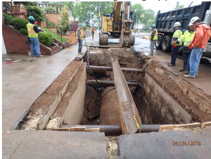
Installation of new water main on 79 th Street (looking west towards Shore Road)
