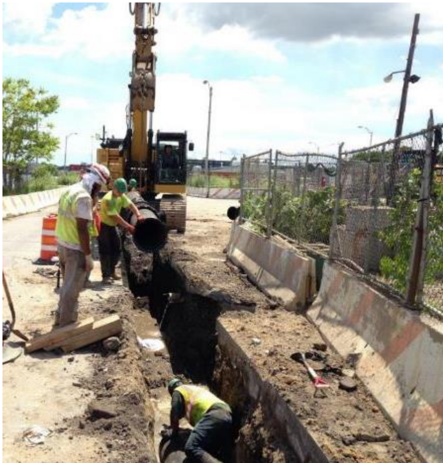
Installation of 20" Water Main along Front Street, looking south
