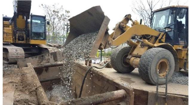
Work related to abandonment of Siphon #1 (at lower Victory Boulevard and Murray Hulbert Avenue), including cutting of pipe and backfilling
