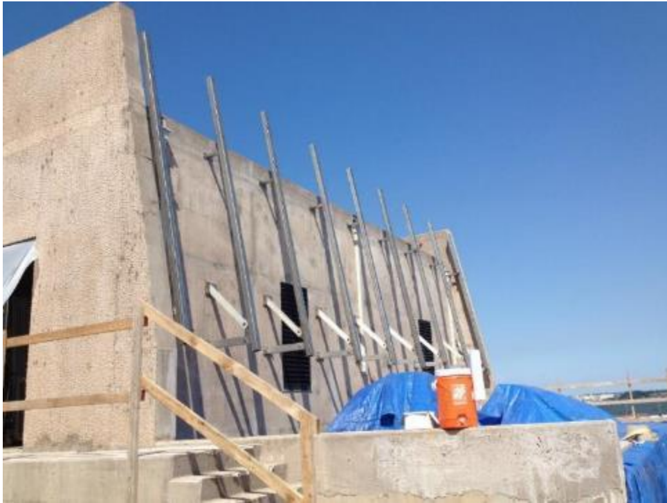
Installation of Chlorination Building Support Frames
