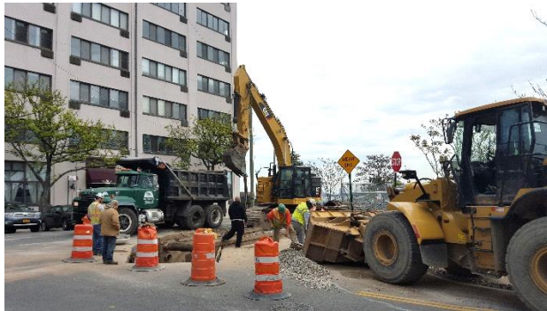
Work related to abandonment of Siphon #1 (at lower Victory Boulevard and Murray Hulbert Avenue), including cutting of pipe and backfilling
