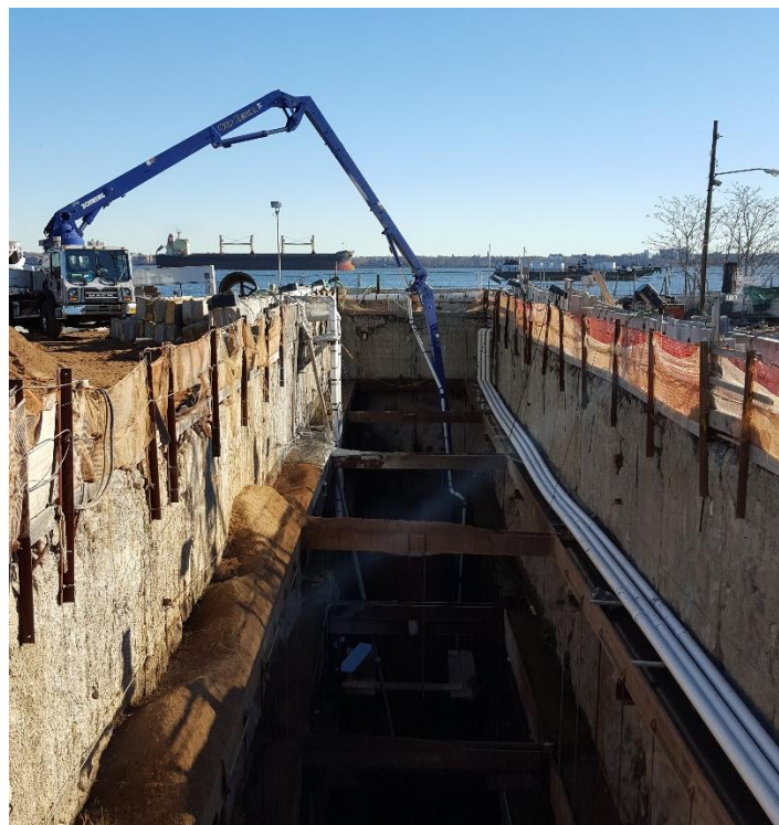
Grouting of riser pipe at Staten Island Shaft Site
