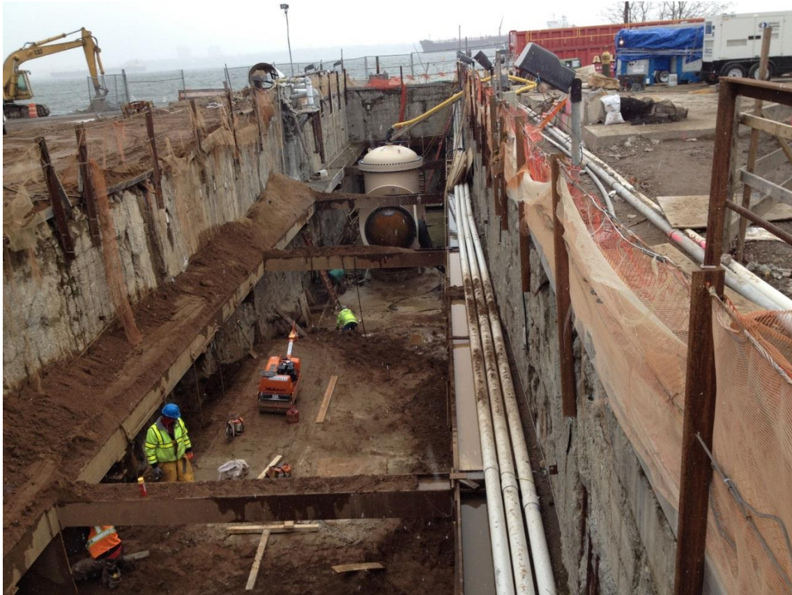
Backfilling of Staten Island Shaft; top of riser pipe is visible in background
