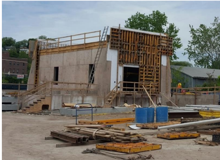
Walls for Chlorination Station at Staten Island Shaft Site begin to take shape
