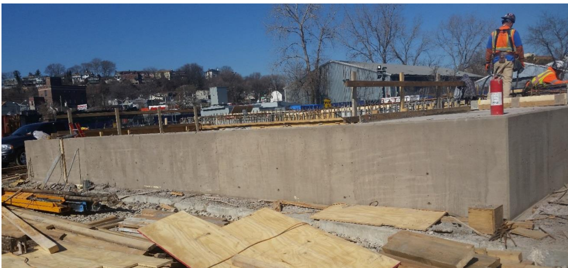
Newly formed exterior wall of Chlorination Station at Staten Island Shaft Site
