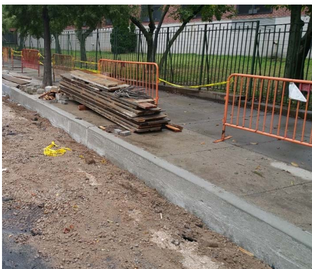
Newly installed curb and sidewalk along Shore Road (in front of Fort Hamilton High School)
