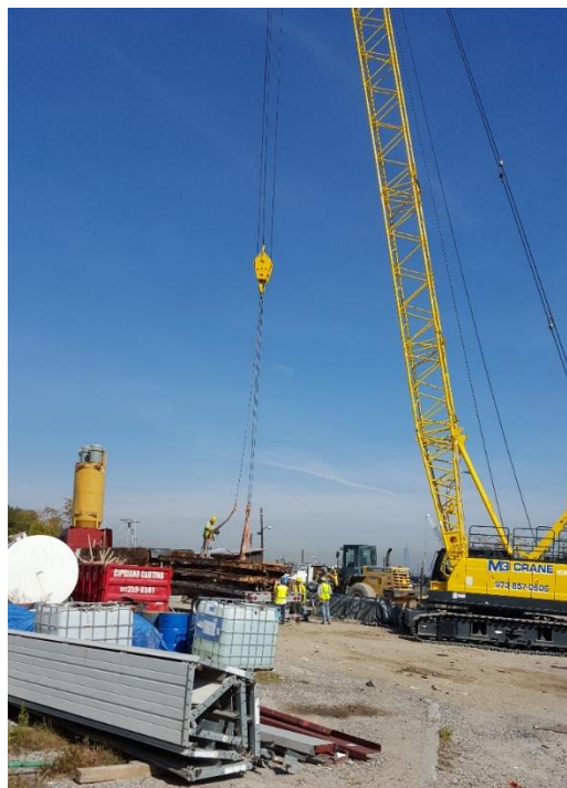
Removal of TBM equipment from the Staten Island Shaft Site.
