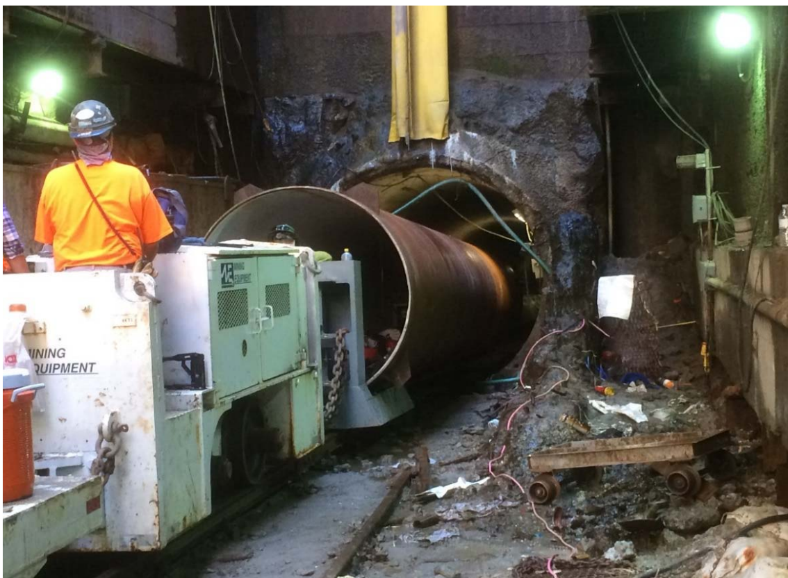
Installation of pipe in tunnel
