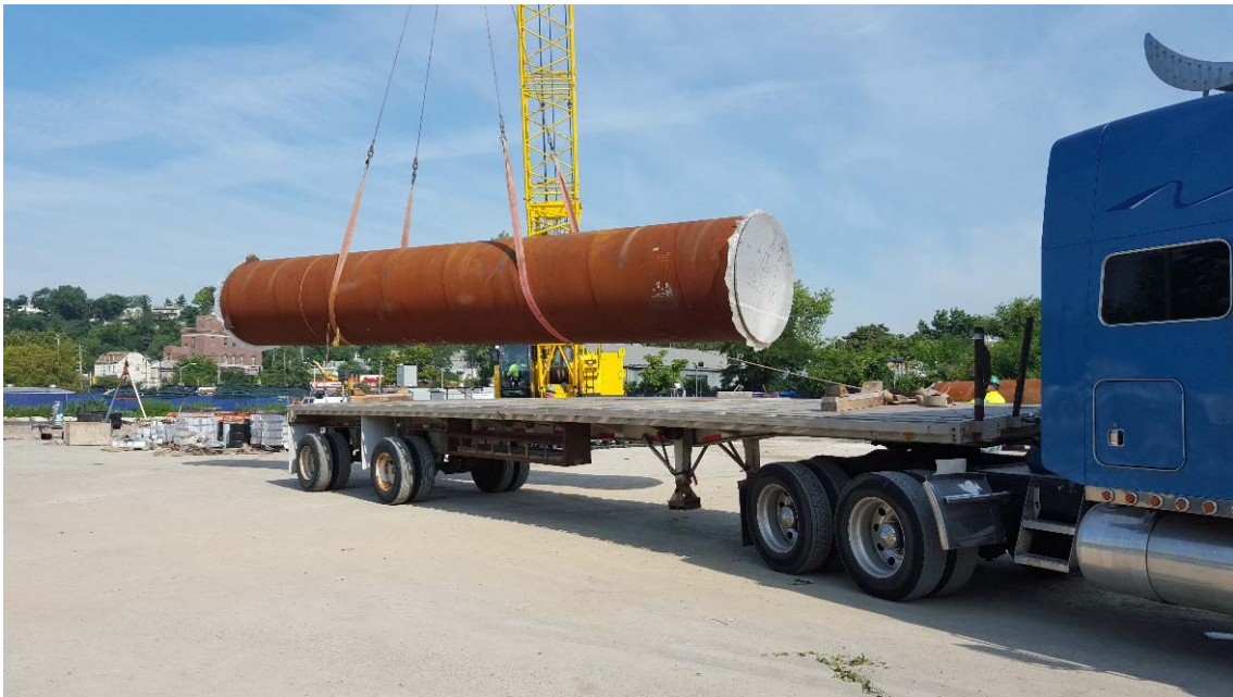
Delivery of 72" carrier pipe for installation in tunnel
