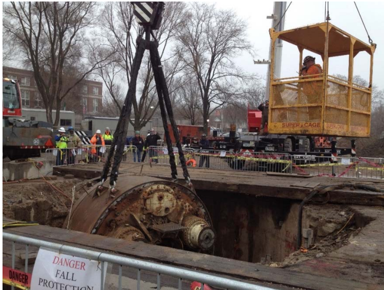
Removal of the TBM cutter head from the Brooklyn Shaft (top and bottom photos)
