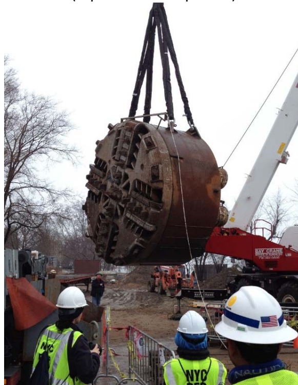
Removal of the TBM cutter head from the Brooklyn Shaft (top and bottom photos)
