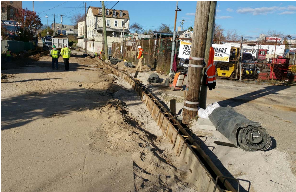
Preparation for installation of new curb along Van Duzer Street, south of Swan Street
