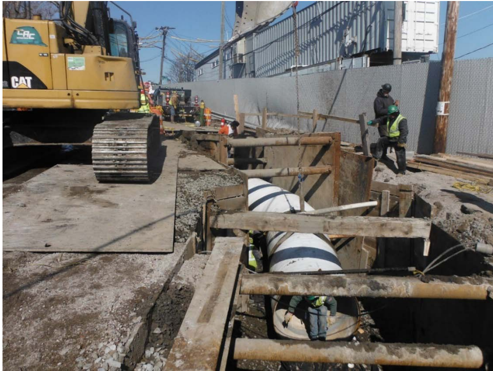
Installation of 60" water main along Front Street, just south of Hannah Street (photo looking north towards Hannah Street)
