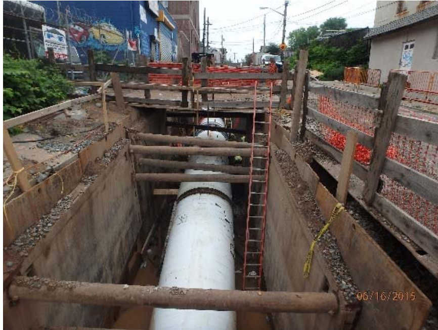
Installation of 72" water main along Van Duzer Street
