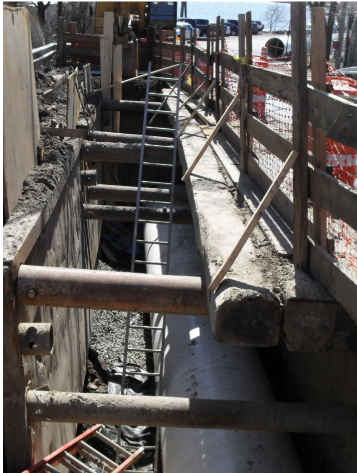
Newly installed 60" water main along Front Street, just south of Hannah Street
