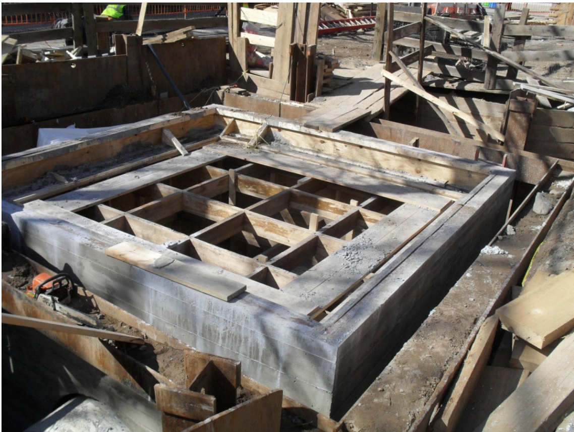
Installation of valve chamber on lower Victory Boulevard
