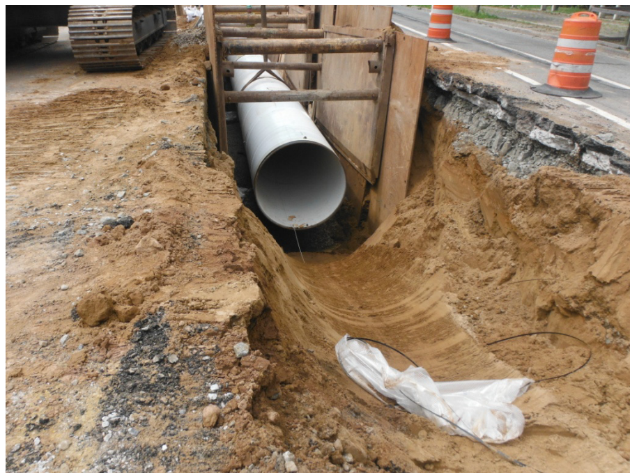
Work related to installation of 72" water main along Shore Road, vicinity of Fort Hamilton High School (top and bottom photos)
