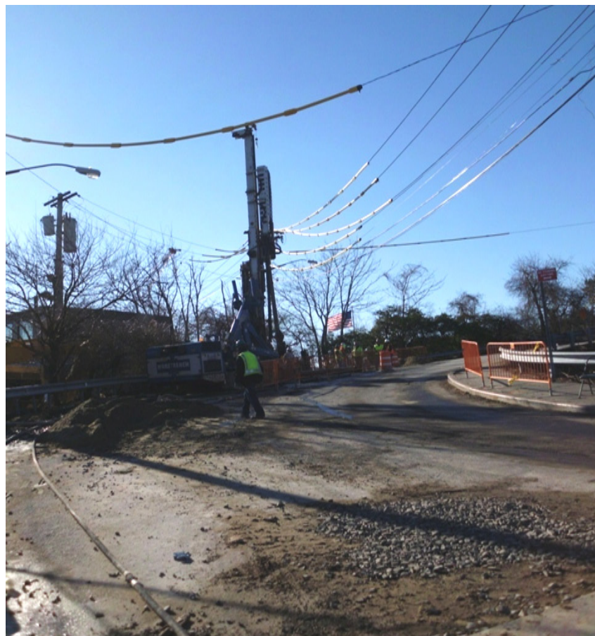
Pile drilling operation on Murray Hulbert Avenue, at Hannah Street
