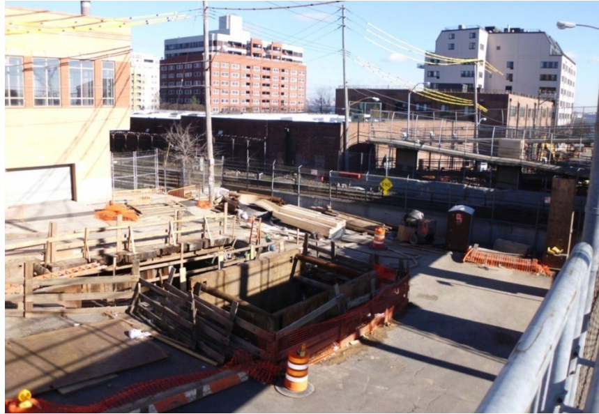
Work related to installation of 60" water main along Victory Boulevard, between tracks and Bay Street
