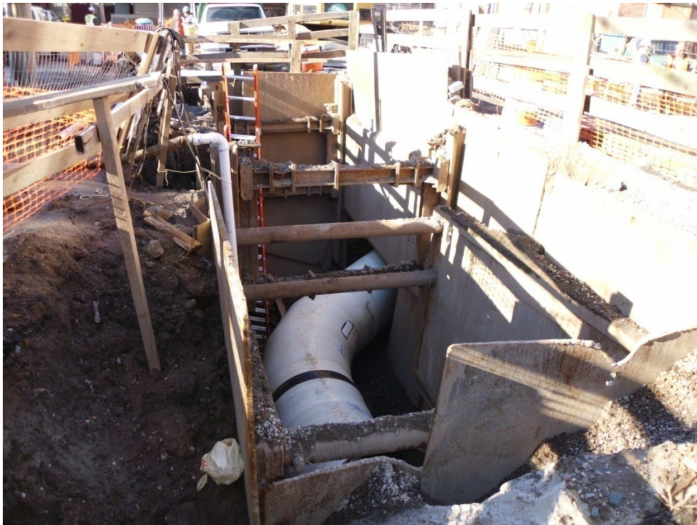
Installation of 60" water main at crossing with 72" sewer (Victory Boulevard, immediately east of tracks)
