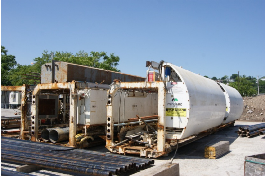
Sections of trailing gear removed from tunnel for repair (top and bottom photos)
