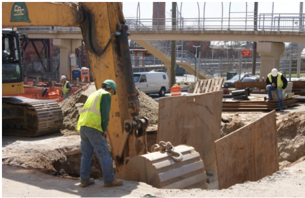
Installation of valve chamber on Victory Boulevard, east of Bay Street
