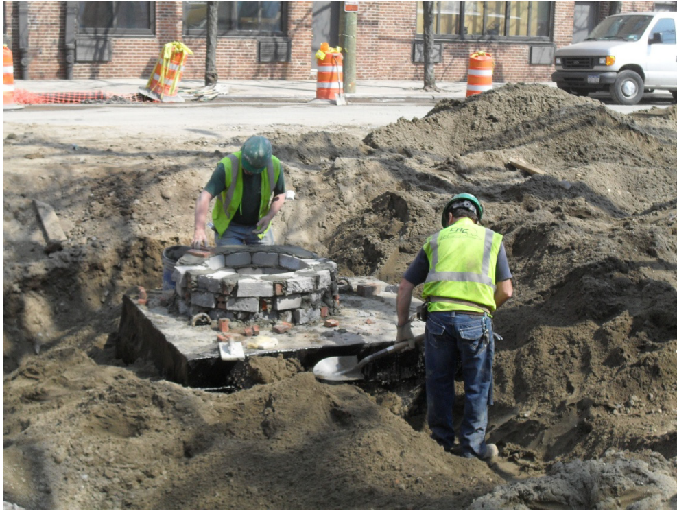
Work related to installation of valve chambers on lower Victory Boulevard (top and bottom photos)
