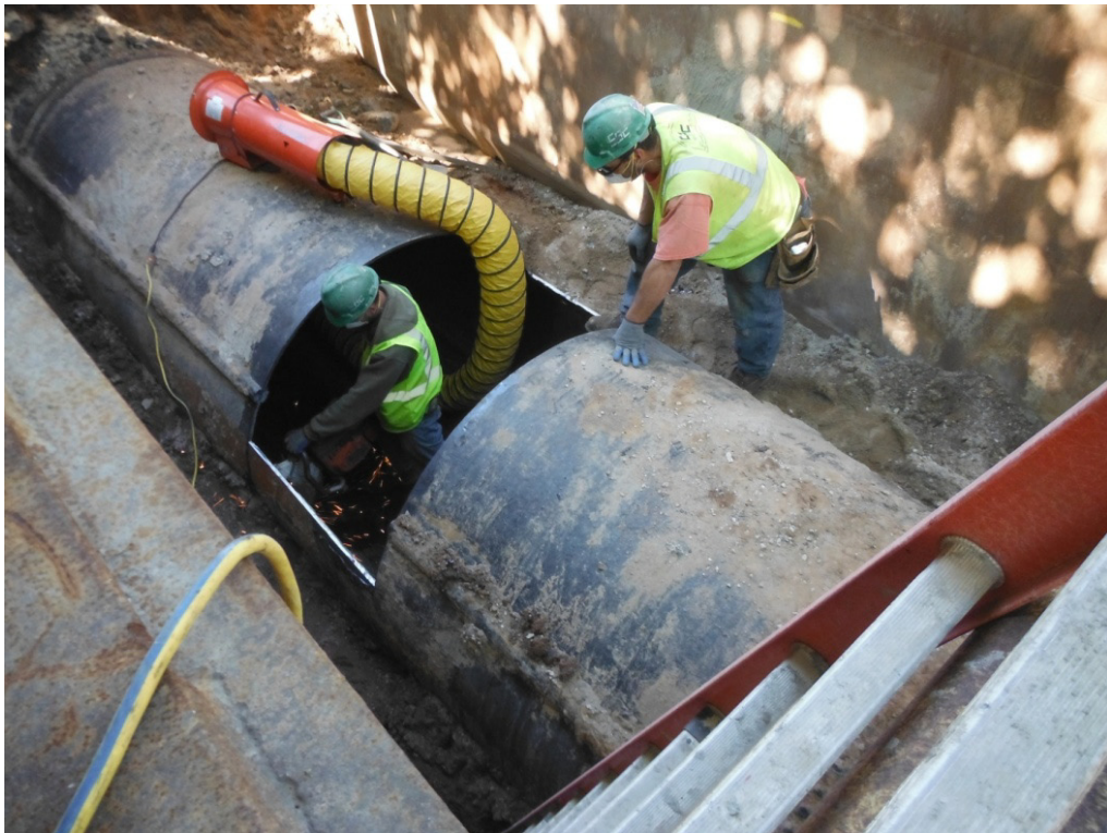
Work related to installation of 60" water main along Shore Road, between 86 th Street and Shore Road Lane (top and bottom photos)
