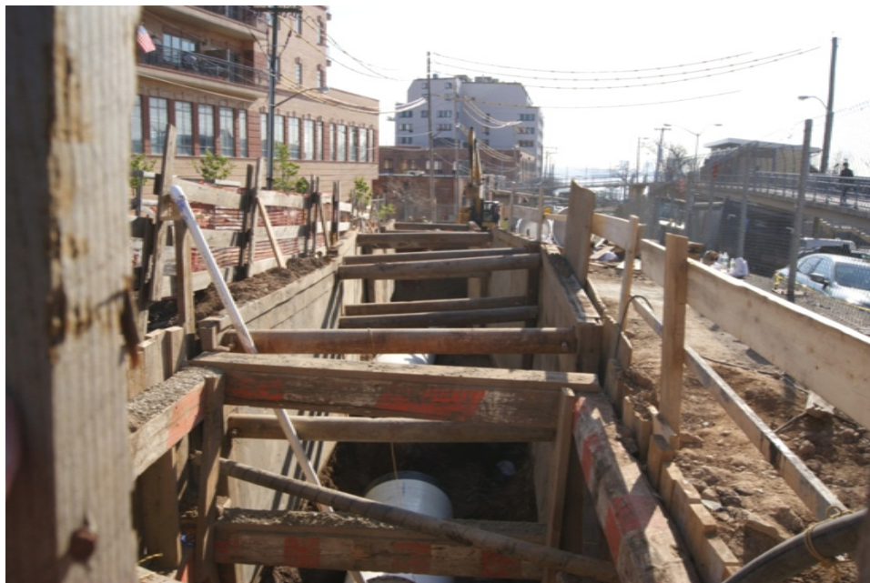
Installation of 60" water main along Victory Boulevard (looking east from Bay Street)
