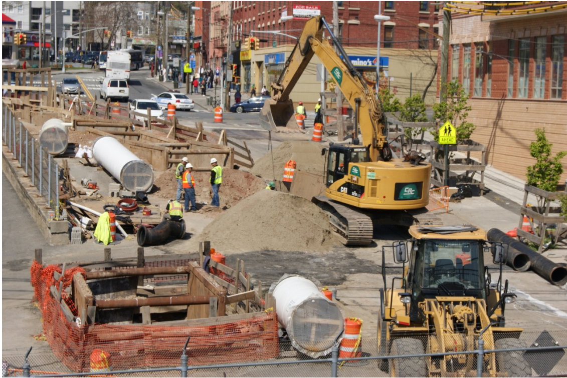
Installation of 60" water main along Victory Boulevard (looking west from Staten Island Railway tracks)
