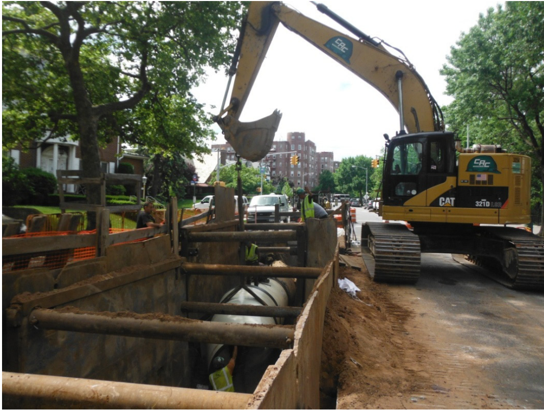
Work related to installation of 60" water main along Shore Road, between 86 th Street and Shore Road Lane (top and bottom photos)
