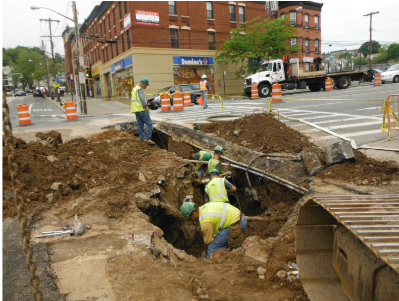
Work related to installation of 12" water main along north side of Victory Boulevard (at Bay Street) (top and bottom photos)
