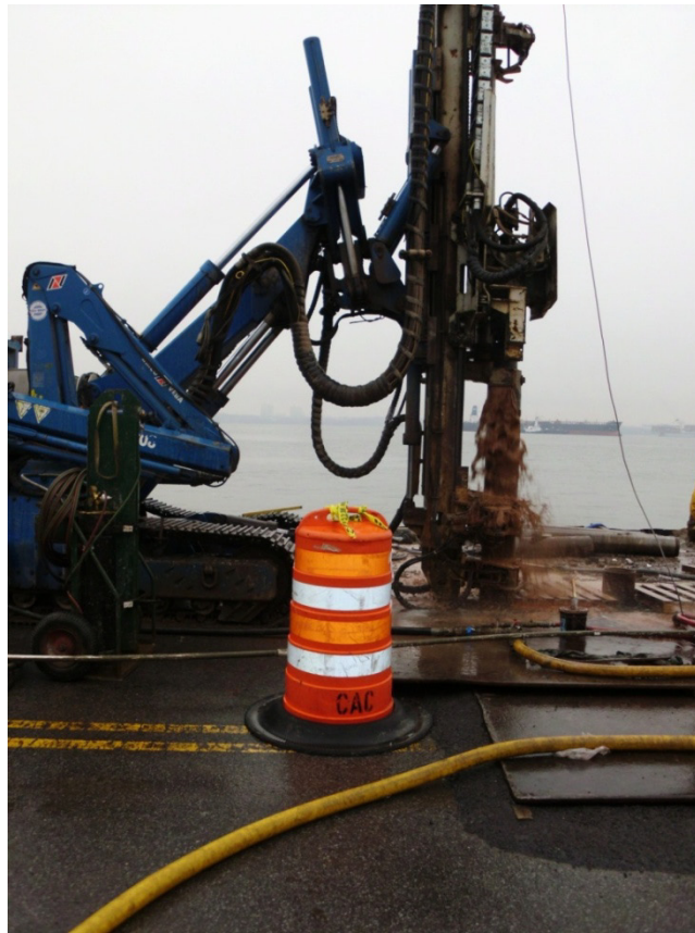
Installation of pile on Front Street, opposite tunnel site
