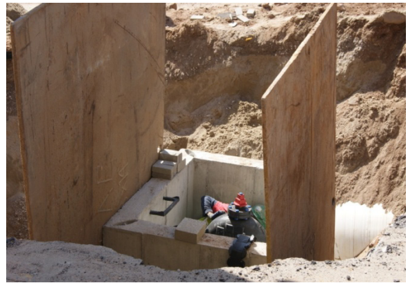
Installation of valve chamber on Victory Boulevard, east of Bay Street
