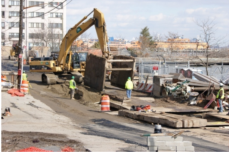
Installation of 60" water main along Murray Hulbert Avenue, looking north towards lower Victory Boulevard
