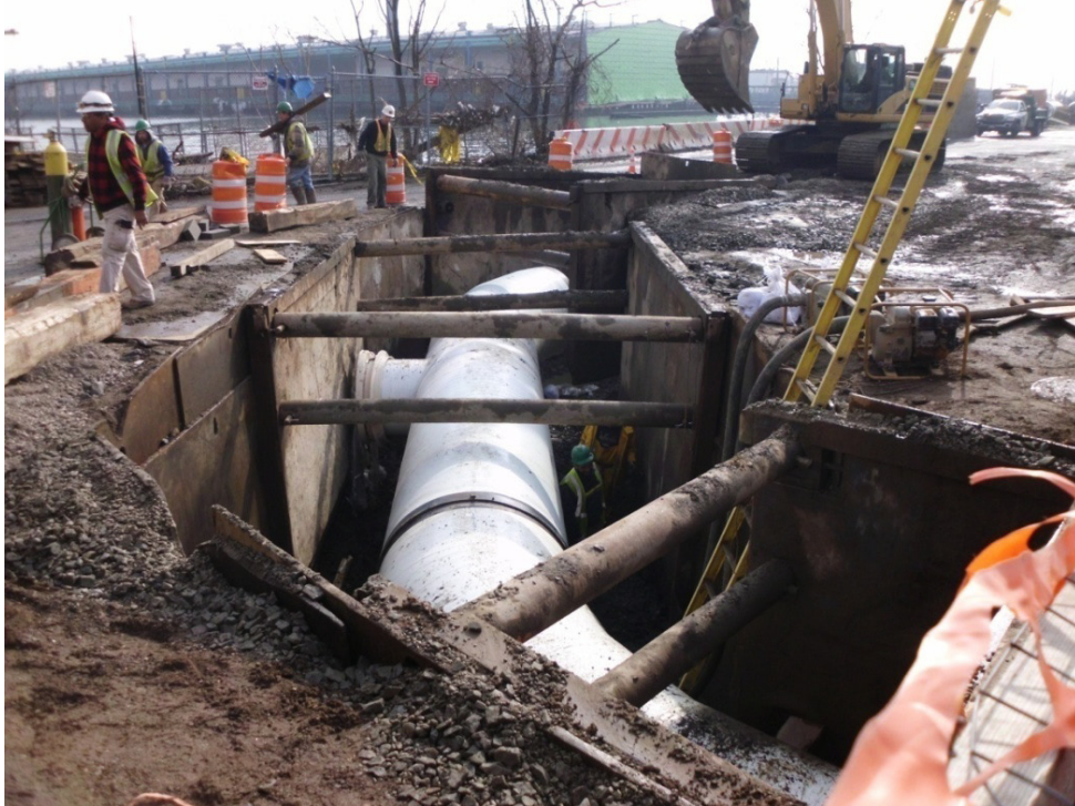
Installation of 60" water main -- proceeding from lower Victory Boulevard towards Murray Hulbert Avenue
