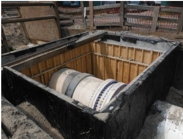
Installation of valve chamber on Shore Road (vicinity of Fort Hamilton High School)
