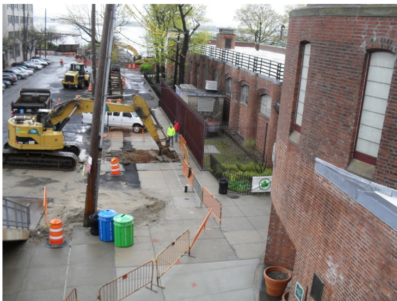
Work related to installation of 20" water main on lower Victory Boulevard
