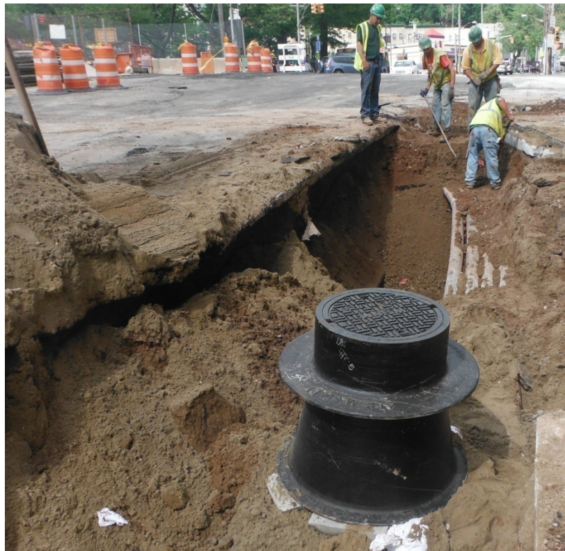
Work related to installation of 12" water main along north side of Victory Boulevard (at Bay Street) (top and bottom photos)
