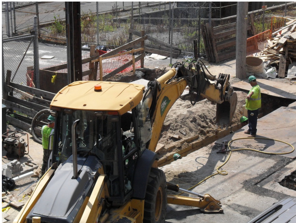
Work related to installation of valve chamber on Minthorne Street, just south of Victory Boulevard
