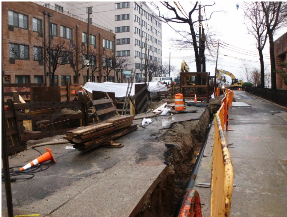
National Grid's gas line relocation work (narrow trench along south side of lower Victory Boulevard, adjacent to 60" water main)
