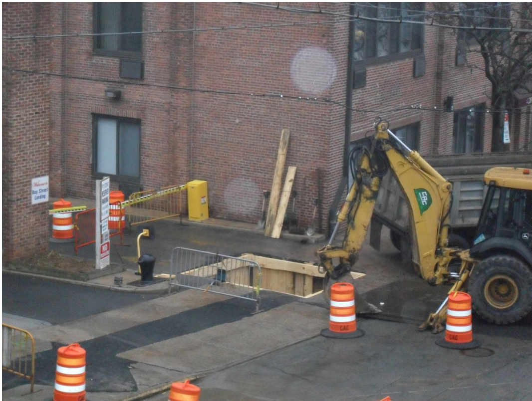
Relocation of gas line (entrance to Bay Street Landing complex, on Victory Boulevard)
