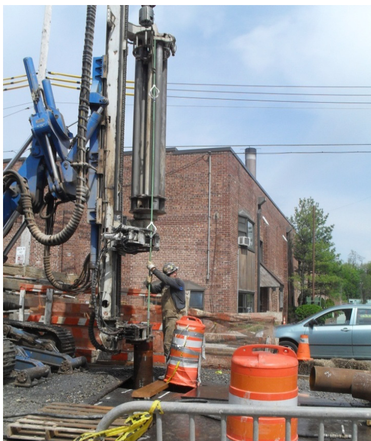
Drilling piles for 24" sewer (Victory Boulevard, just east of SIRR tracks)
