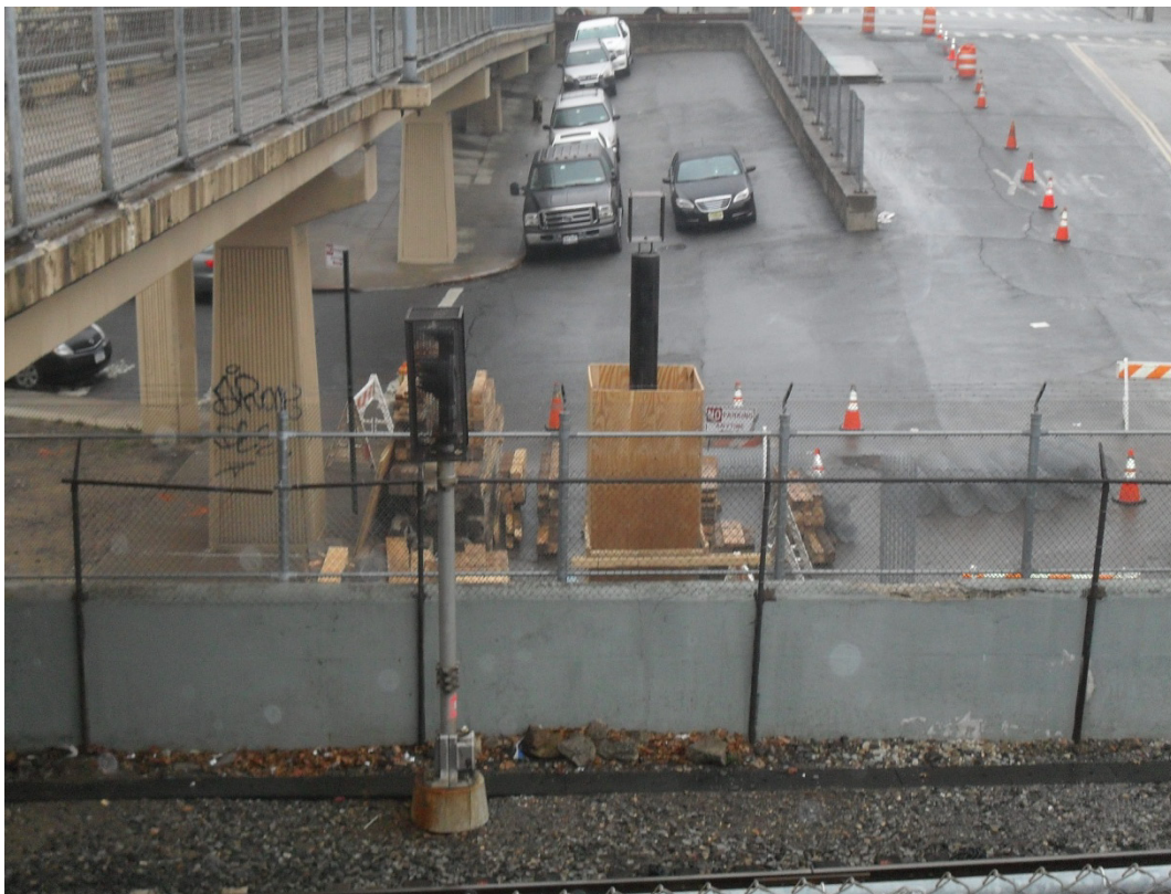
Installation of pole for monitoring system along Staten Island Railroad at Victory Boulevard
