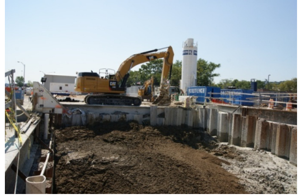
Foundation of new Chlorination Station, which is being used as a muck pit during tunnel excavation
