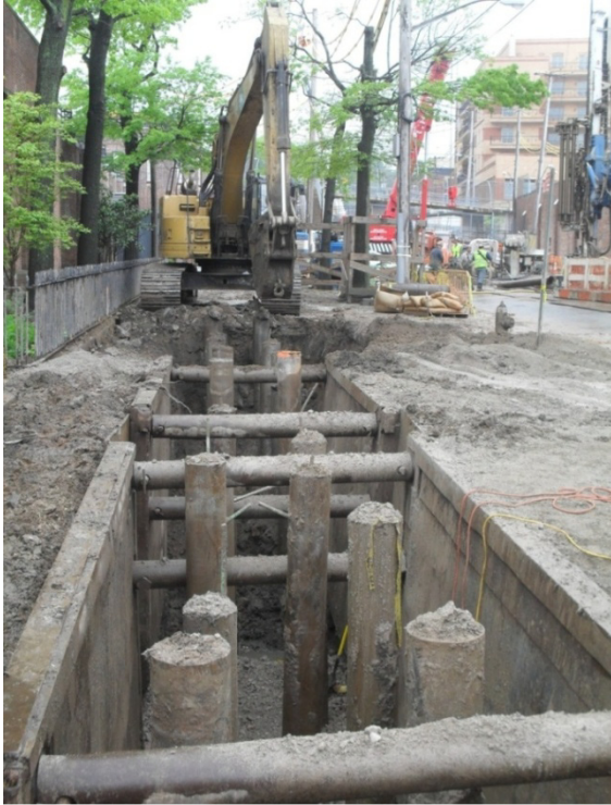
New piles along south side of Victory Boulevard, east of SIRR, in preparation for installation of 24" sewer
