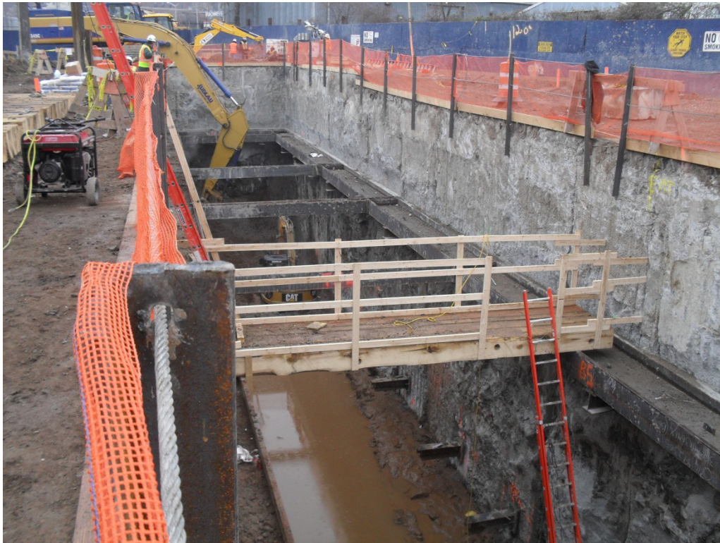
Excavation of starter trench at Staten Island shaft site
