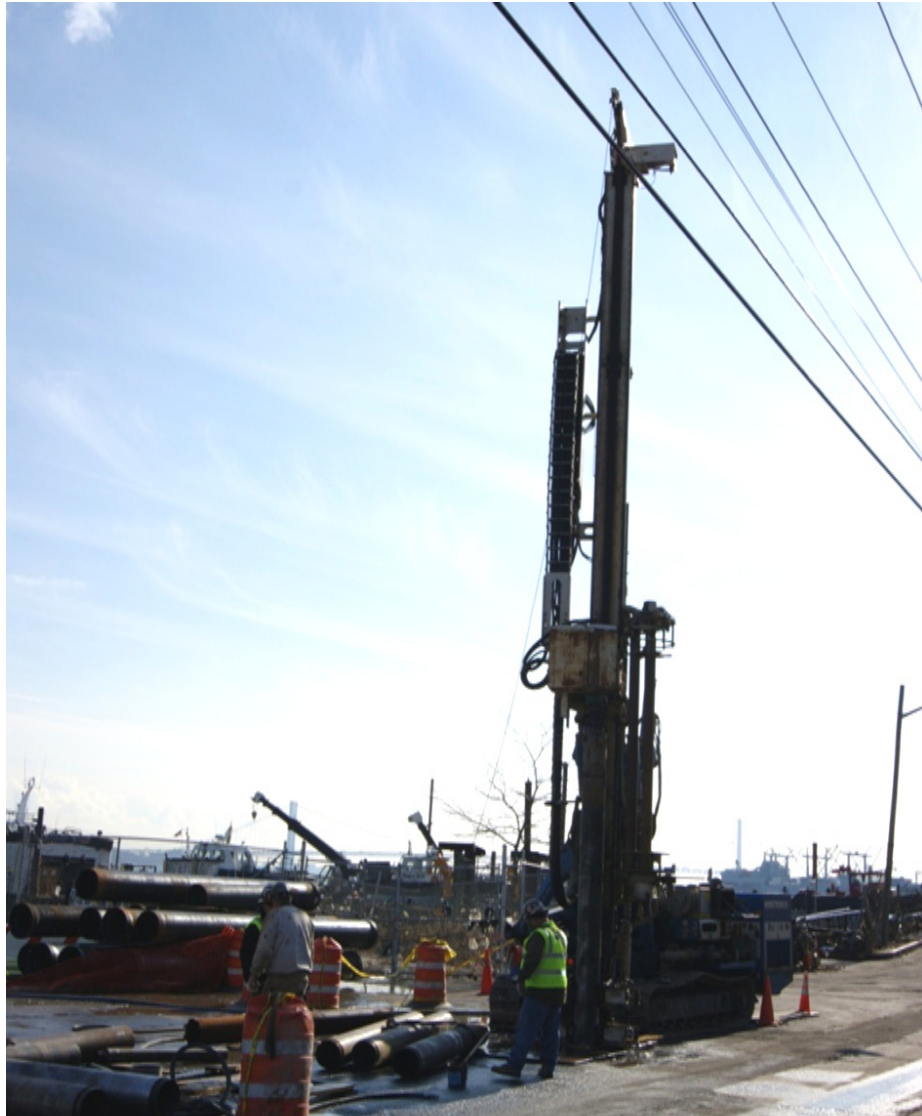
Pile drilling operation on Murray Hulbert Avenue, between Victory Boulevard and Hannah Street
