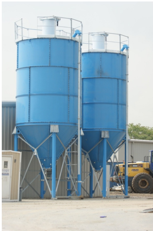
Grout plant at starter trench in Staten Island
