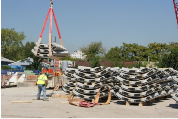
Ring segments being lifted for placement in starter trench
