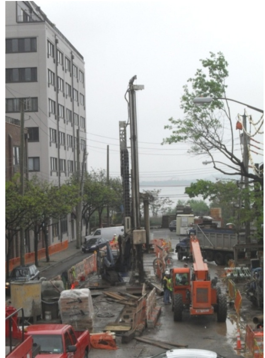
Installation of piles for 72" sewer along Victory Boulevard, east of SIRR
