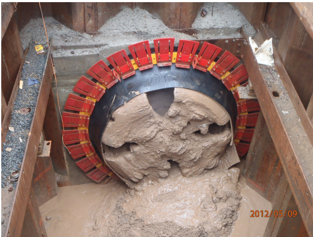
Microtunneling “break through” beneath SIRR tracks on May 9, 2012 (Victory Boulevard, east of SIRR tracks)
