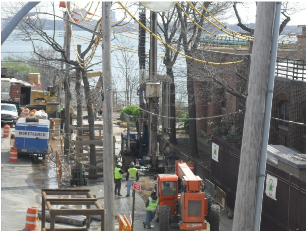
Installation of piles for 24" sewer (along Victory Boulevard, adjacent to Lyons Pool)
