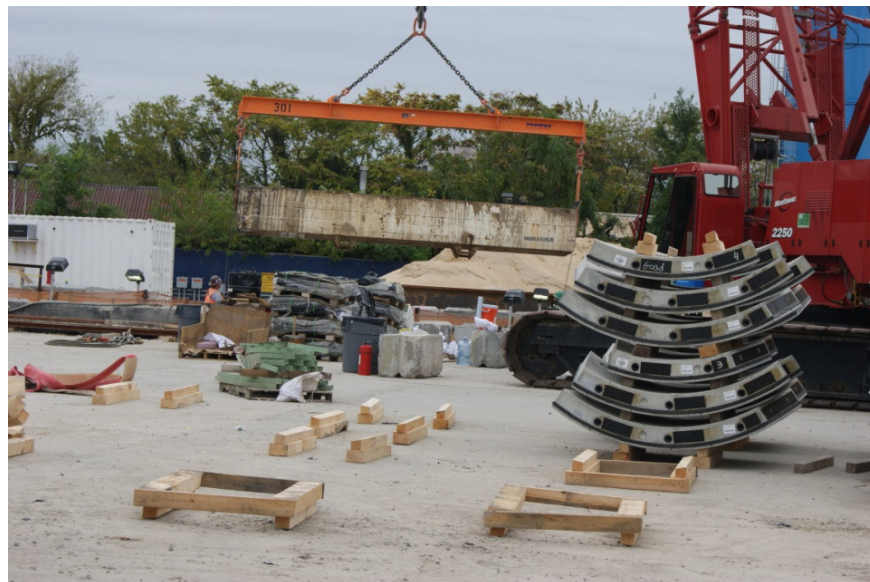
Removal of muck car from trench; precast segment rings in foreground (at right)
