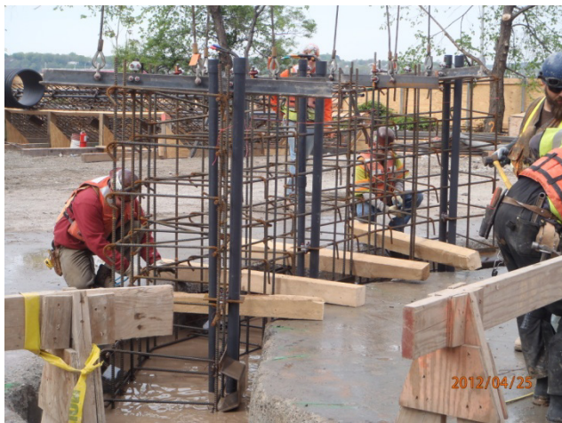
Assembly of panel for Brooklyn slurry wall
