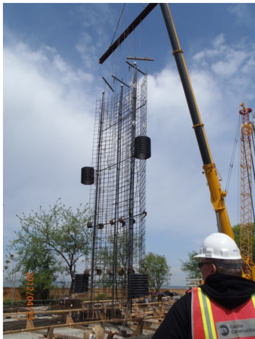
Slurry wall panel being placed at Brooklyn shaft site
