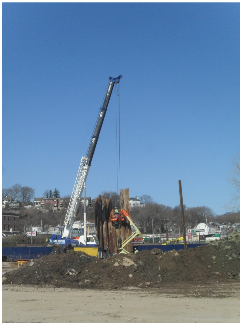
Installation of sheeting for jacking pit (in yard near starter trench, east side of SIRR tracks)
