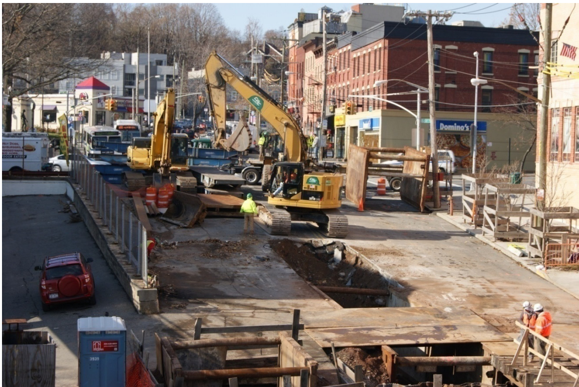
Excavation for 60" water main along Victory Boulevard (looking west towards Bay Street)
