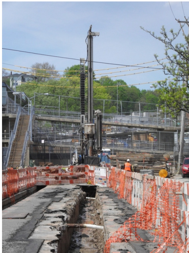
Excavated trenches in preparation for pile drilling for installation of 72" sewer (Victory Boulevard, east of SIRR)
