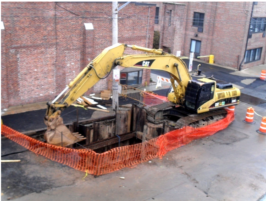
Installation of jacking pit, Victory Boulevard just east of SIRR tracks
