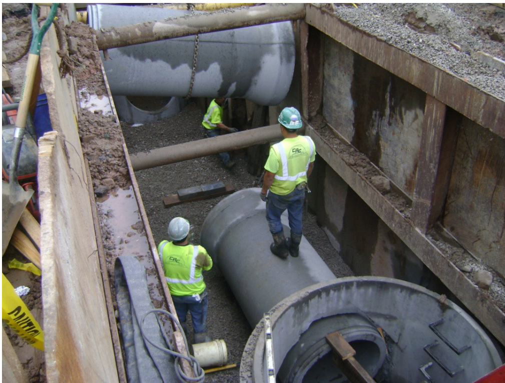
Installation of 36" sewer along Shore Road, between 86 th Street and Shore Road Lane
