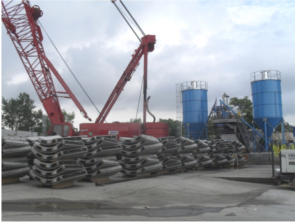
Sections of precast segment rings prior to installation in tunnel
