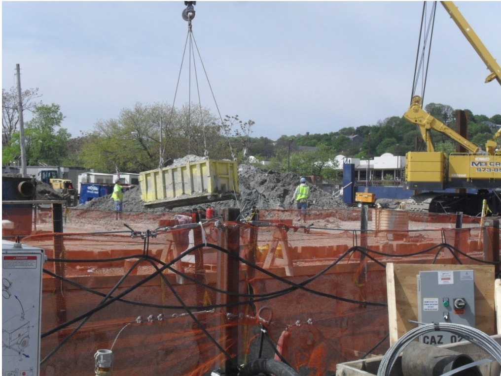
Removal of excavated material from starter trench in Staten Island
