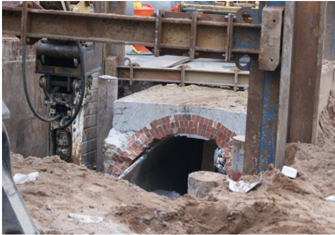
Replacement of 72" sewer beneath Victory Boulevard, east of SIR tracks (photo at left: removal of existing 72" sewer) (photo at right: installation of new sewer)
