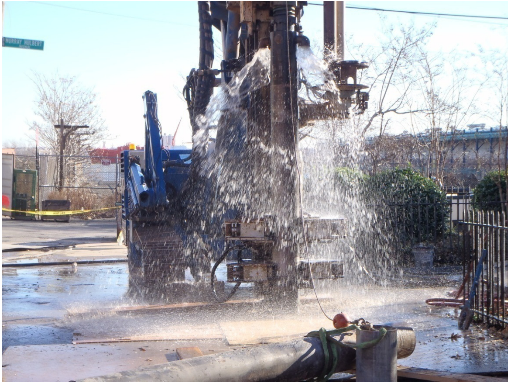
Drilling of casing pipe in preparation for placement of test piles (intersection of Murray Hulbert Avenue and Victory Boulevard)
