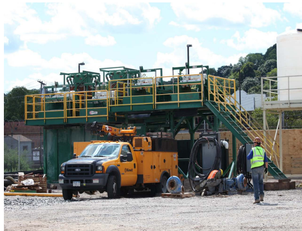
Equipment used to recycle slurry material for reuse during installation of panels
