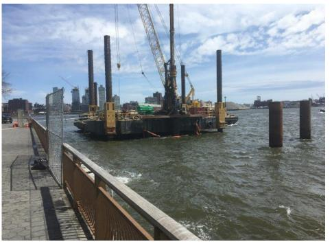
Barge mounted drill rig
